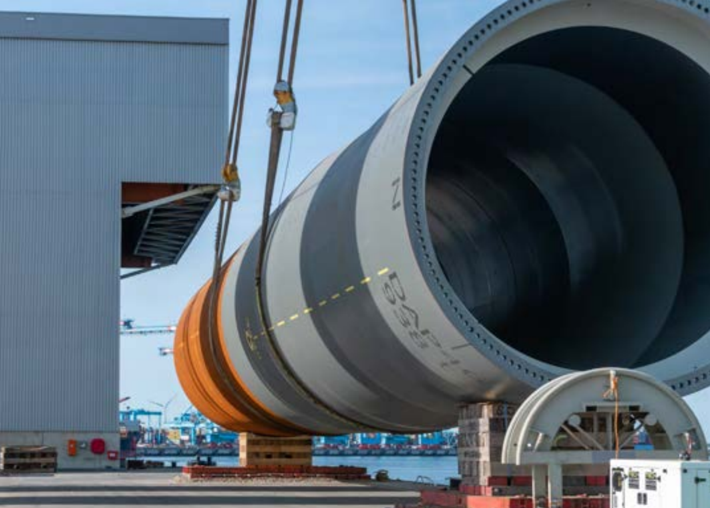
The load out of a monopile
