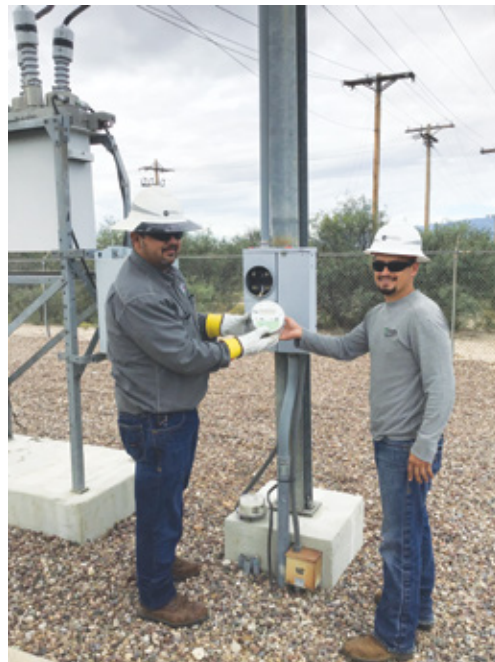
Jesus Moreno and Reggie Martinez install the last single-phase meter
