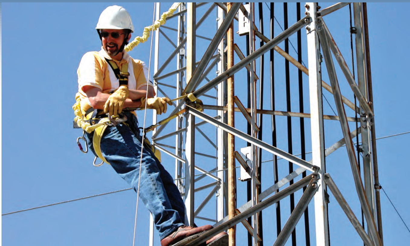
FAA technician working on a communication tower.
