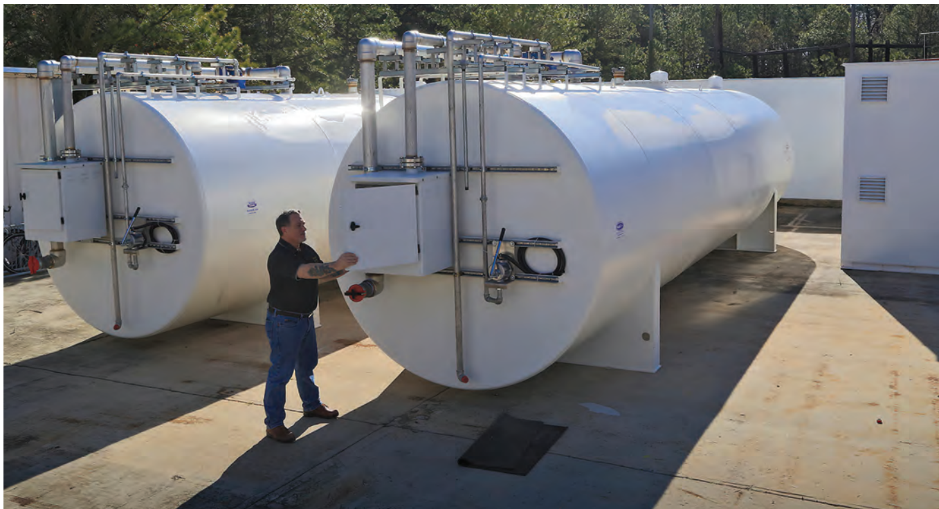
Twin 10,000 gallon tanks used for alternative fuel testing at the William J. Hughes Technical Center's Propulsion and Airpower Engineering and Research Lab.
