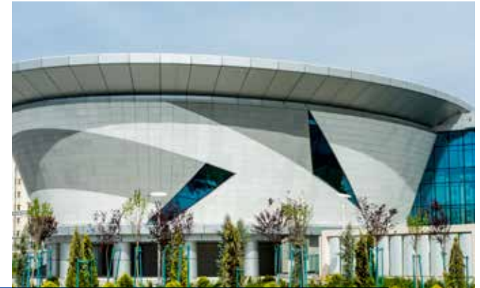
Ashgabat Simple Cycle Power Plant
