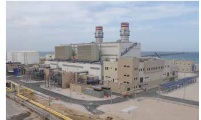
Al-Khums Simple Cycle Power Plant
