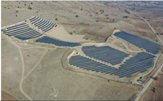
Taşova Solar Power Plant
