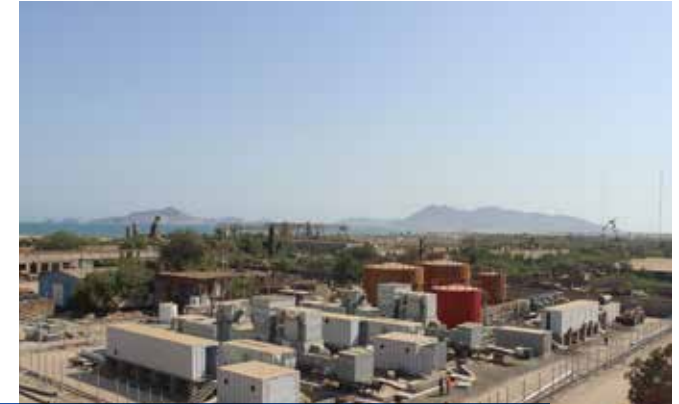
Aden Simple Cycle Power Plant
