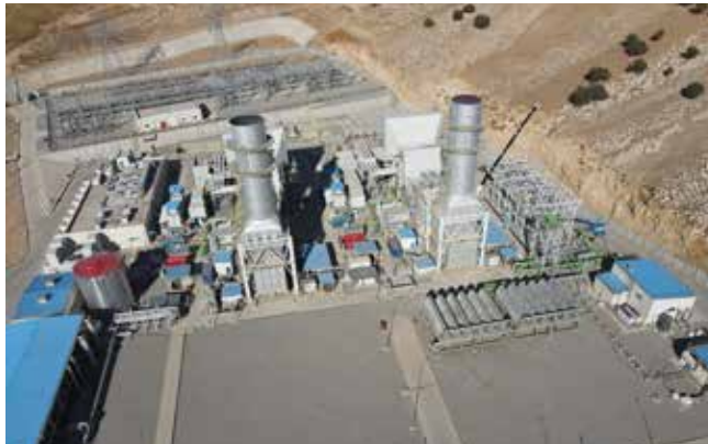
Bazian Simple Cycle Power Plant
