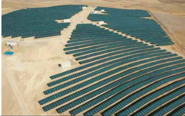
Erzincan Solar Power Plant
