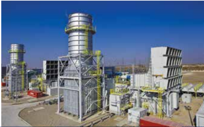
Ahal-2 Simple Cycle Power Plant
