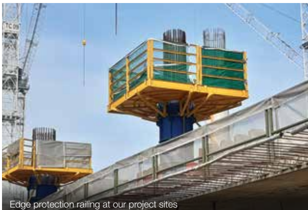
Edge protection railing at our project sites
