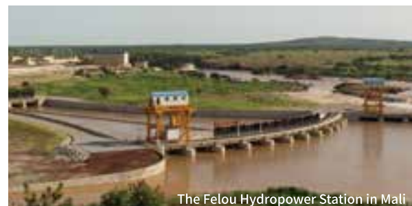
The Felou Hydropower Station in Mali
