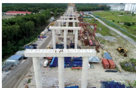
Completed column and cross heads at Tanjung Pelepas area
