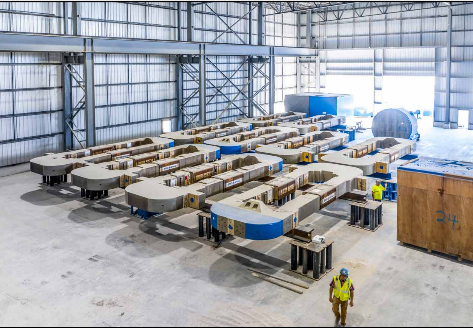
Each of the mill stands for SDI weighs 160 tons. —
