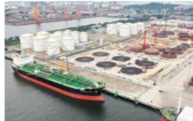
Aerial view of Jurong Port Tank Terminals
