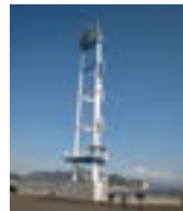
津波待避所を備えた照明塔 Lighting tower equipped with tsunami shelter
