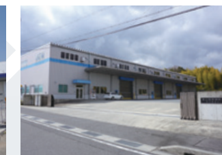
Kuwana Distribution Center
