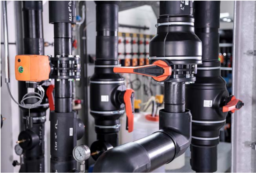
COOL-FIT 4.0 enables reliable and safe cooling for industrial and commercial systems with 30% higher energy efficiency.
