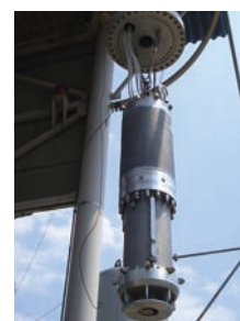
Installation of cryogenic pump
