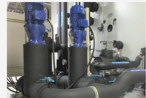
Installing the modified wet film reduces the rinsing water pump's energy consumption by 80%
