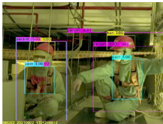
Hazard Analysis for Ceiling Maintenance - Using AI to detect if workers are wearing safety helmets and safety harnesses
