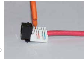
2. Placing the keystone jack on the fixture and setting the wire pairs on IDC according to the wiring configuration A or B.
