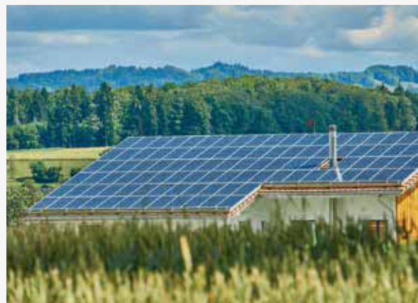
Photo: SolarX installation.
