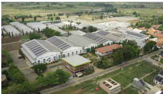
Indonesia: solar rooftop installation. © Xurya Daya Indonesia.
