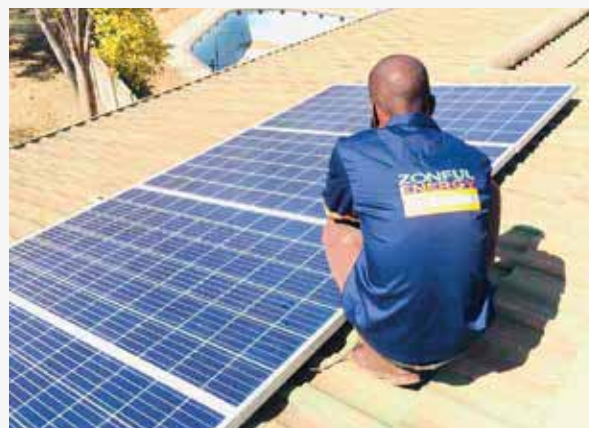
Photo: Zonful; solar panel installation.
