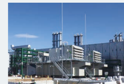
Gunma Complex (Gunma Prefecture), which is increasing its electricity self-sufficiency by adding gas turbines for power generation
