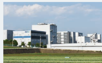
Yokonodaira Plant at the Gunma Complex (Gunma Prefecture, Japan), where capital investment to expand capacity is underway.
