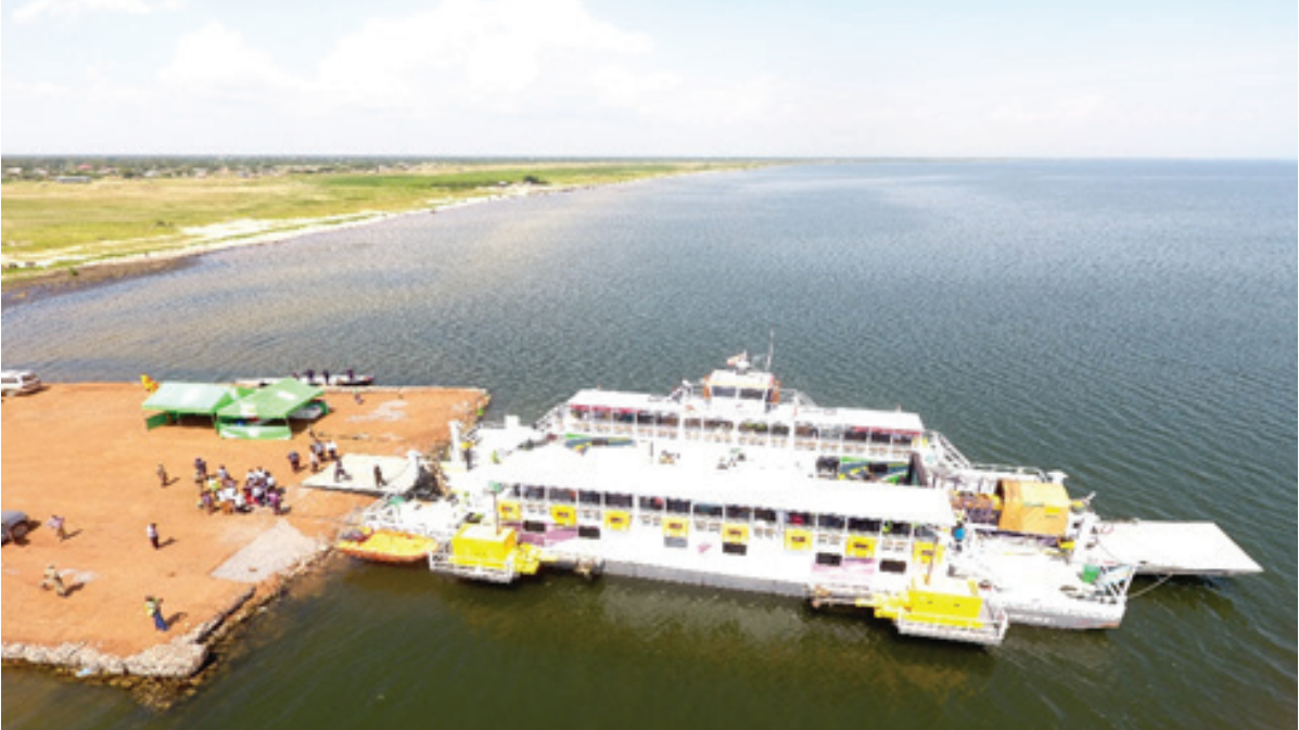
Figure 12: The new Kyindi-Buvuma Ferry (above) connects Kiyindi and Buvuma and MV Albert Nile1 (below) connect Panyimur to Wanseko
