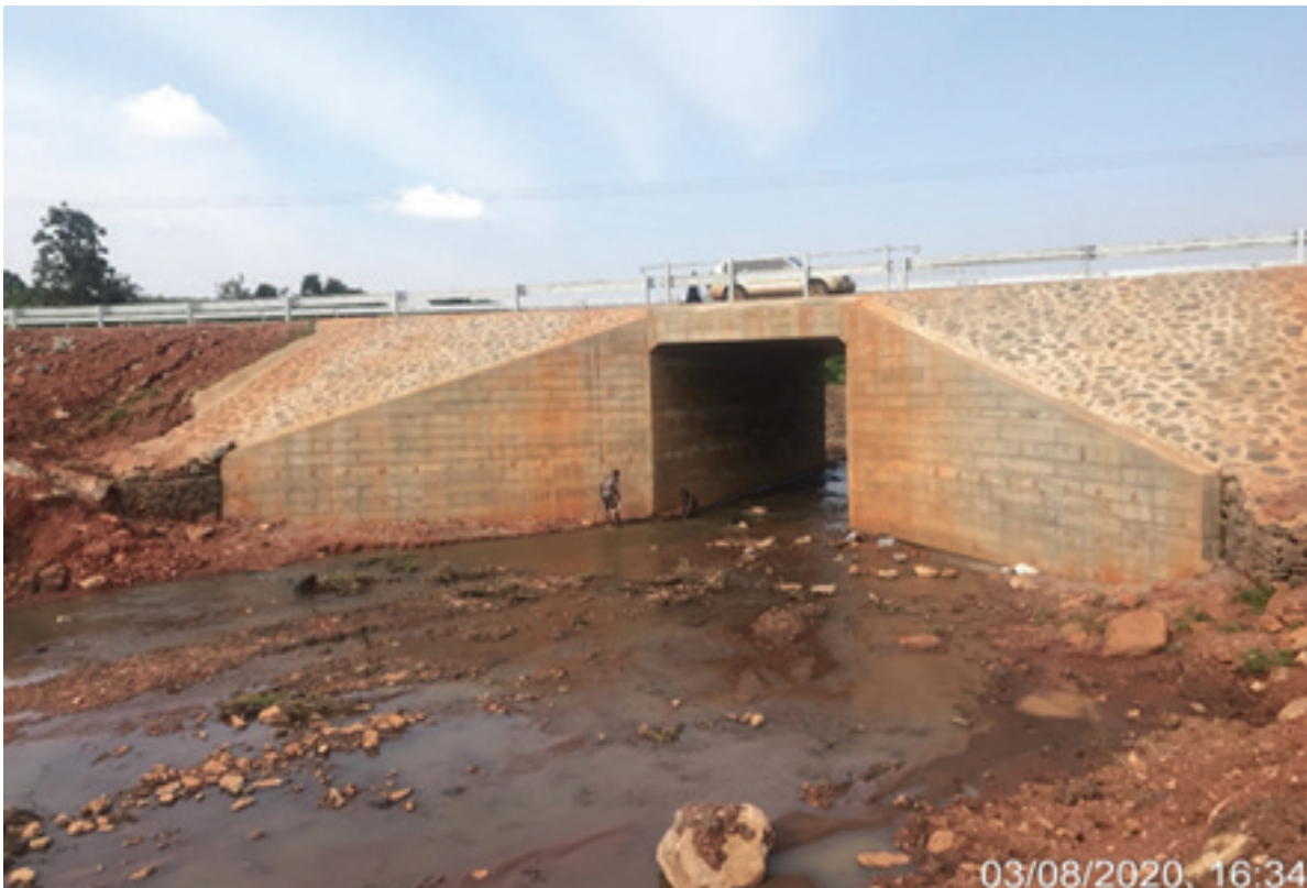
Figure 11: Nsongi Bridge (above) and Wakiri Bridge (below)
