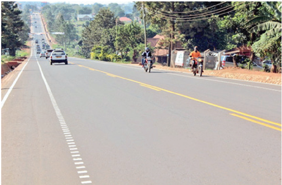
Figure 10: Fort Portal - Kyenjojo Road (above) and Hima-Katunguru rehabilitation projects(below)
