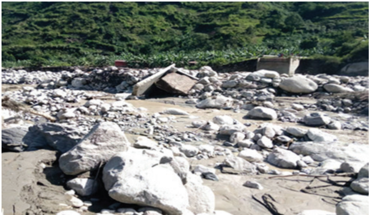
Figure 5: Section of Kasese - Kilembe road (above) and Kyanjuki Bailey Bridge (below) washed away by heavy rains
