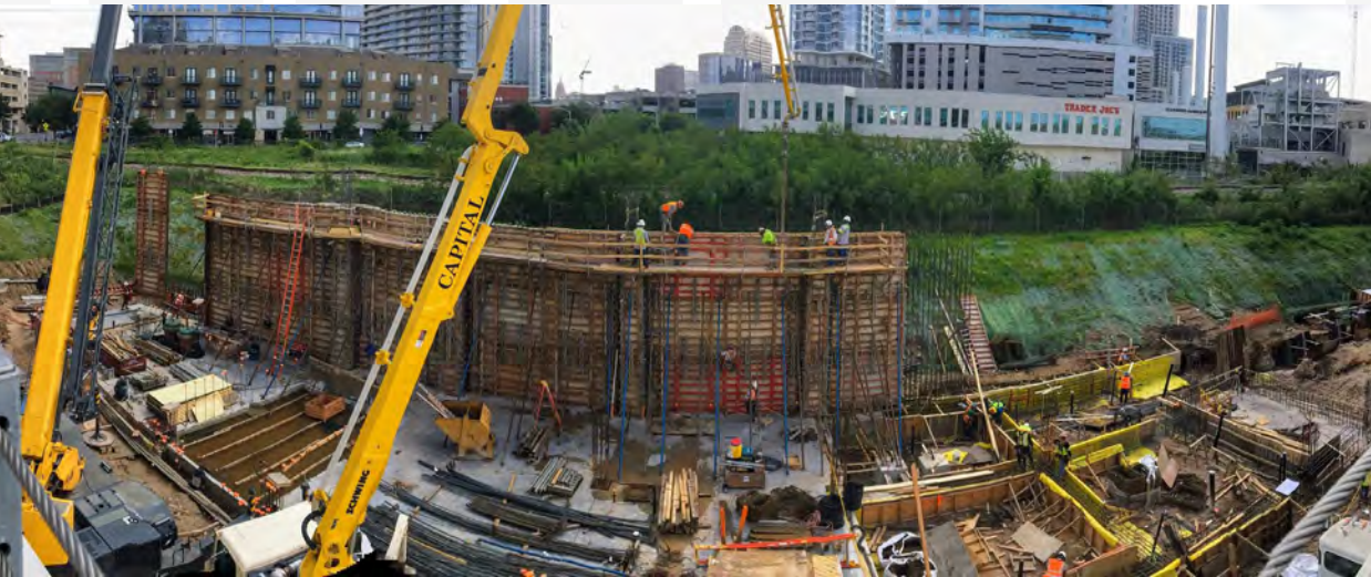
In 2019 District Cooling Plant #3 (DCP3), located in the Seaholm eco-district, moved into a second year of construction. Crews completed much of the concrete shell for both buildings and the underground piping necessary to add 10,000 tons of capacity to the downtown cooling loop. DCP3 will be completed in 2020.
